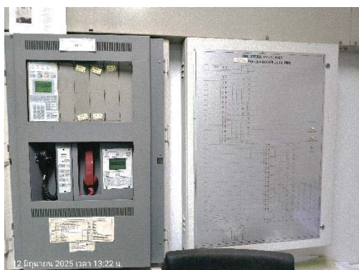
Fire Alarm Control Panel : FCP
